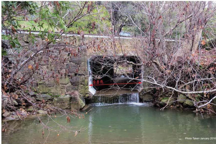
Figure 26. KVP-5 - Existing Condition at Stonybrook Creek Culvert, seen from south of SR-84
