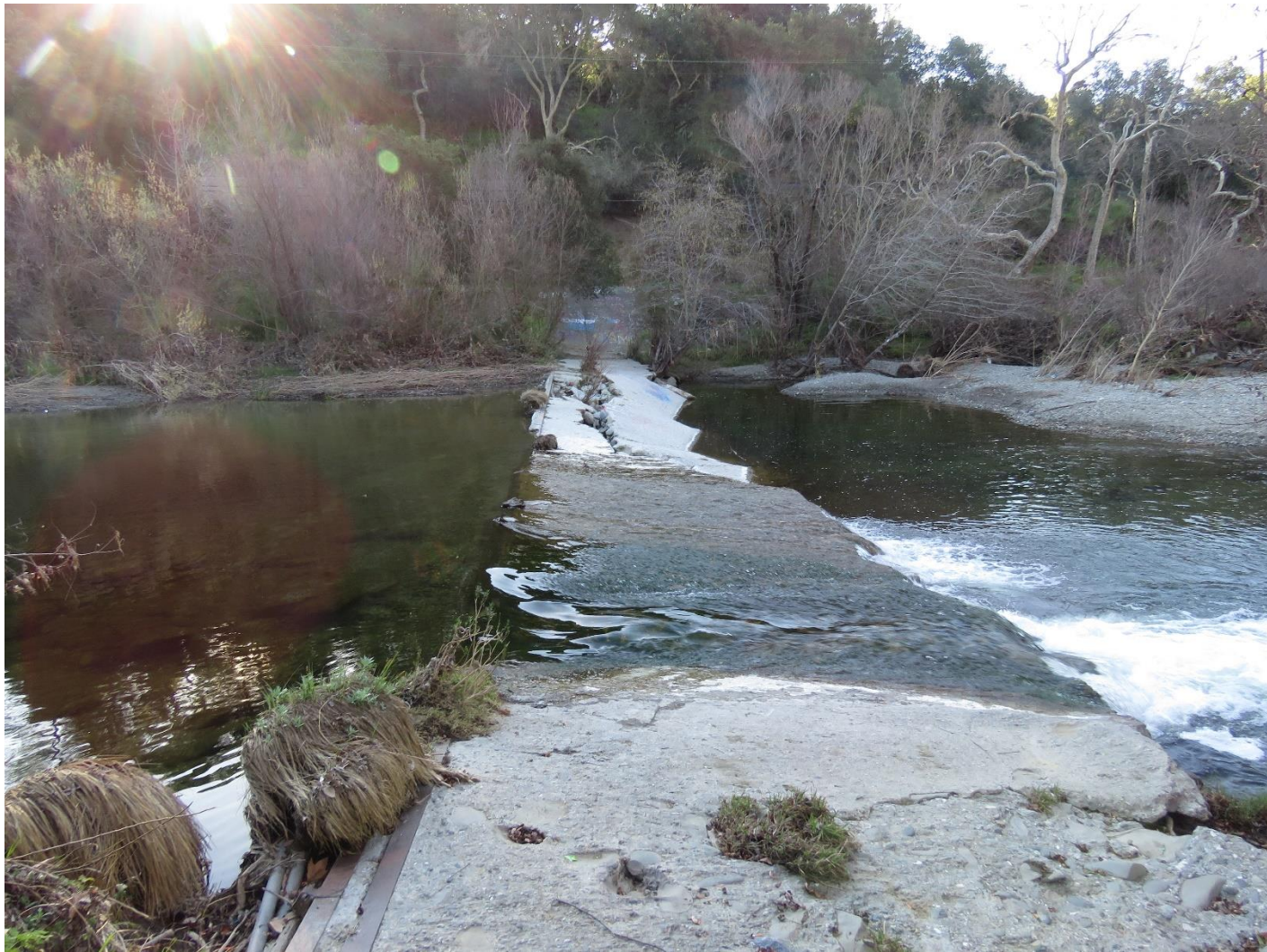
Failing Cement Apron at USGS Gaging Station
