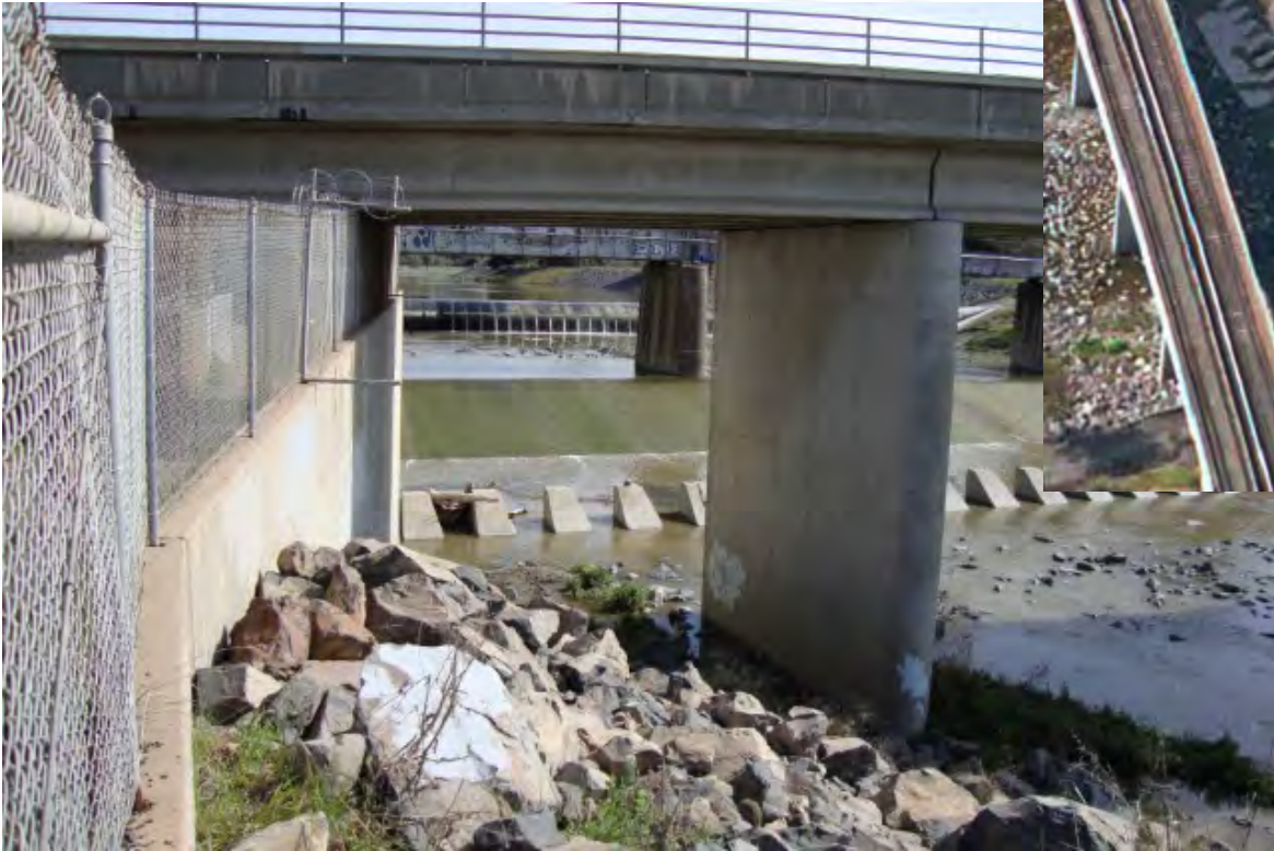
Drop Structure looking up at RD1
