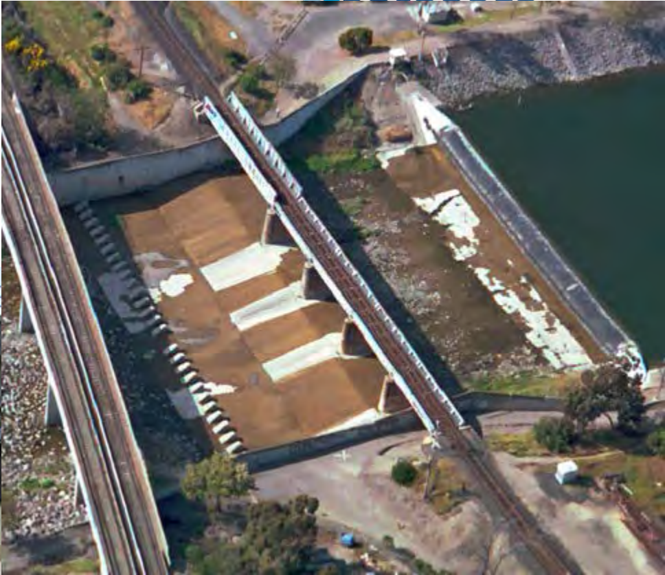
RD1/Drop Structure aerial
